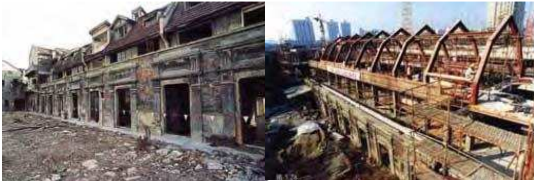
Figure 7.4. The original appearance of stone gate row and the new roof frames added in the renovation work of Shikumen houses.
