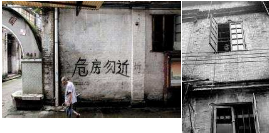
Figure 8.1. Dangerous and dilapidated buildings
