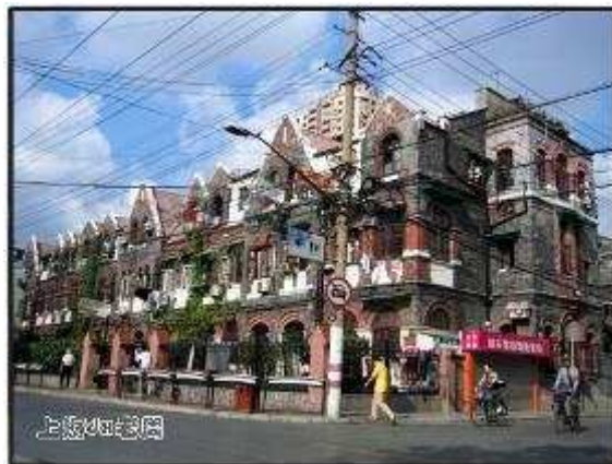
Figure 7.8. Historical heritage buildings in the area (舟山路, Zhou Shan Road)
